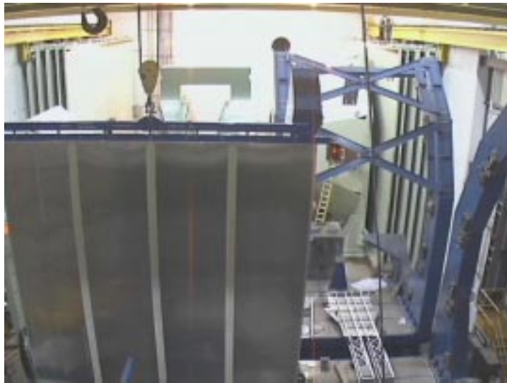
Figure 3: A large panel being installed into the PHENIX Experimental Hall.
